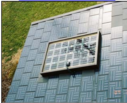
4'x6' integrated photovoltaic glass is used as a skylight over the Pool House, 14W Atlantis Sunslates as roofing.
