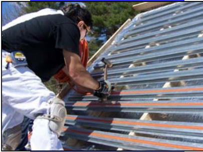
Installing the solar thermal tubing below the Atlantis Energy Sunslates
