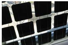
Siemens 4 x 4-inch solar cells laminated with clear low-e. Design by Adrian Smith, SOM Chicago.
